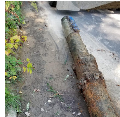
SW Garden View Drive pipe replaced during main break in 2022.
