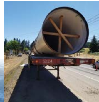
This is pipe from our neighbors at Tualatin Valley Water District as they build a new water source, state-of-the-art water filter treatment plant, and transmission line to bring Willamette River water into eastern Washington County.
