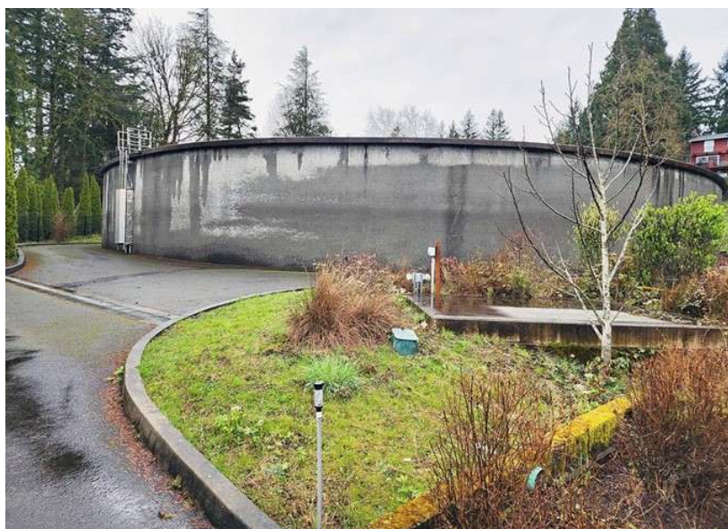
Reservoir #3 at Sylvan Hill, completed in 2009.
