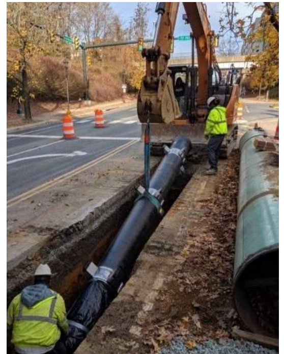
Construction worker installing water main in street.
