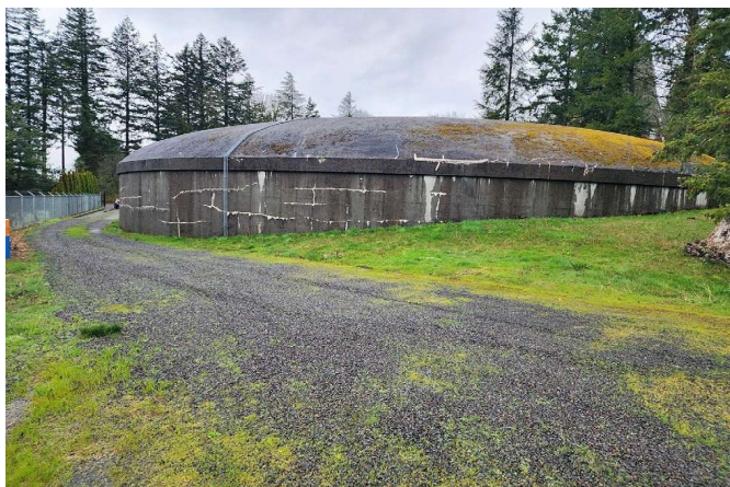
Picture of the District's Reservoir #2 (2.25 MG of storage), built in 1961 and not earthquake resilient.
