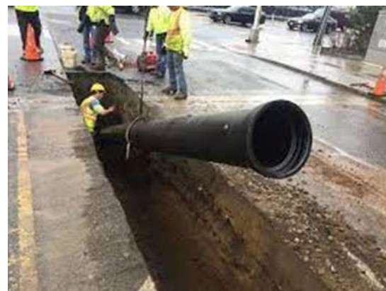
Construction crew installing water main pipe.
