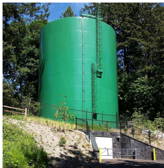
The District's Green Tank on Canyon Drive.
