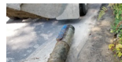
District staff work on leak at SW Canyon Drive.
