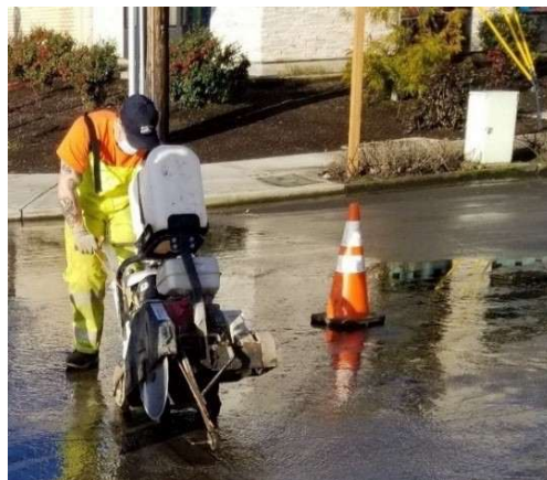
District staff saw cutting street for pipe project.
