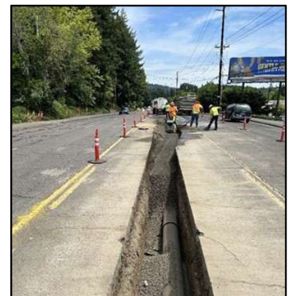
Beaverton-Hillsdale main pipe replacement project, showing trench for pipe installation.
