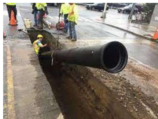
Construction crew installing water main pipe.
