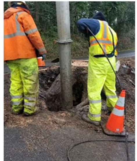
District staff drilling in the street to remove tree root.
