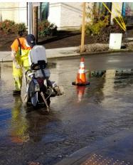
very good condition. But as water mains age, they become susceptible to breaking. When a main breaks, we cut through the pavement, dig a hole to find the leaking pipe, and put a repair band
