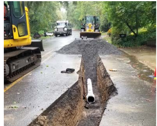
Pipe trench on SW Garden View Avenue
