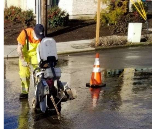
District staff saw cutting street for pipe project.
