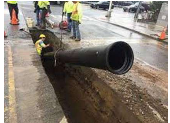
Construction crew installing water main pipe.
