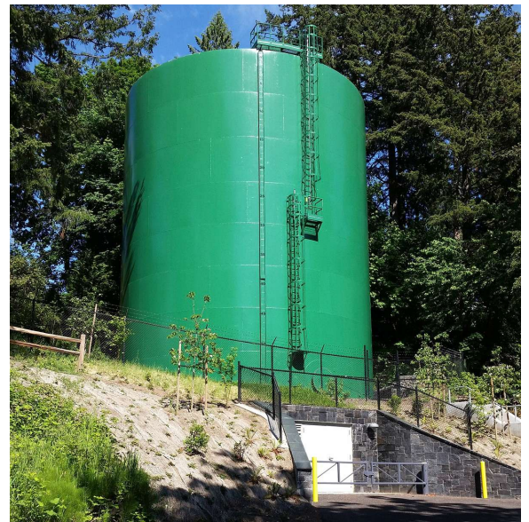
The District's Green Tank on Canyon Drive.
