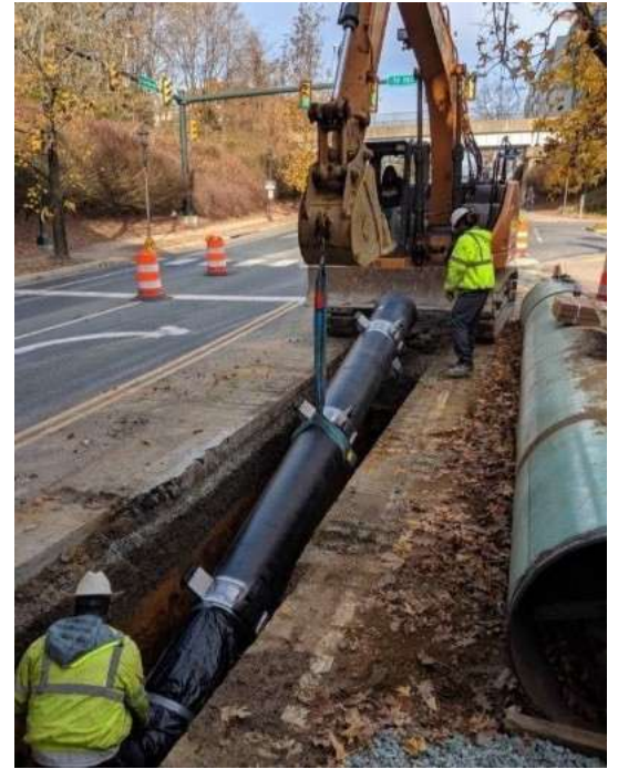
Construction worker installing water main in street.
