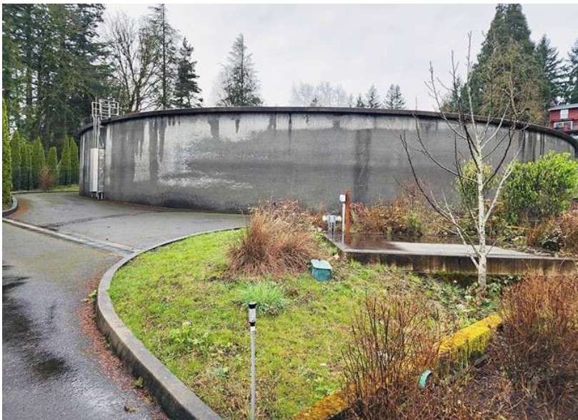
Reservoir #3 at Sylvan Hill, completed in 2009.
