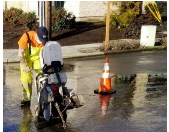
District staff saw cutting street for pipe project.
