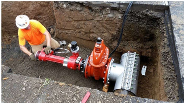
Construction worker connecting into water main pipe.
