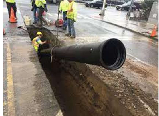
Construction crew installing water main pipe.
