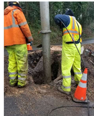
District staff drilling in the street to remove tree root.
