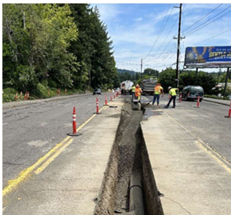
Beaverton-Hillsdale main pipe replacement project, showing trench for pipe installation.
