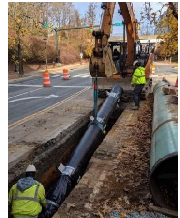
Construction worker installing water main in street.
